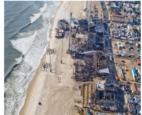
Destructive Boardwalk fire in 2013.
